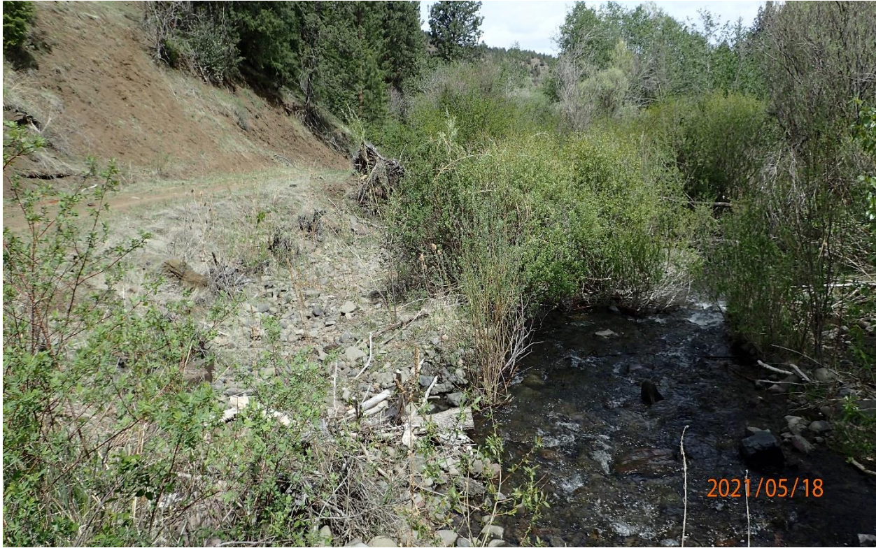
Above: Overview of bank stabilization and vegetation.
