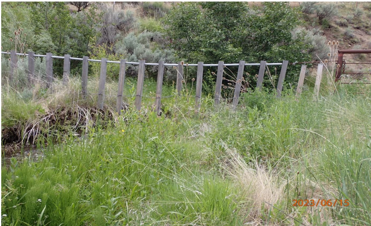
Below: Upstream from bridge, after instream grade control riffles were installed.
