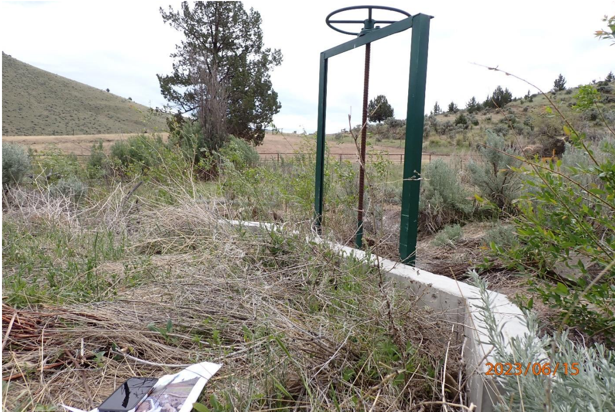
Above: After project completion. Showing large woody structures, HD fencing, new diversion, and riparian plantings.
