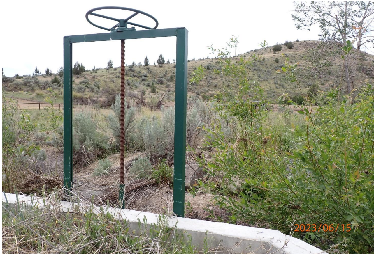
Above: New diversion structure.
