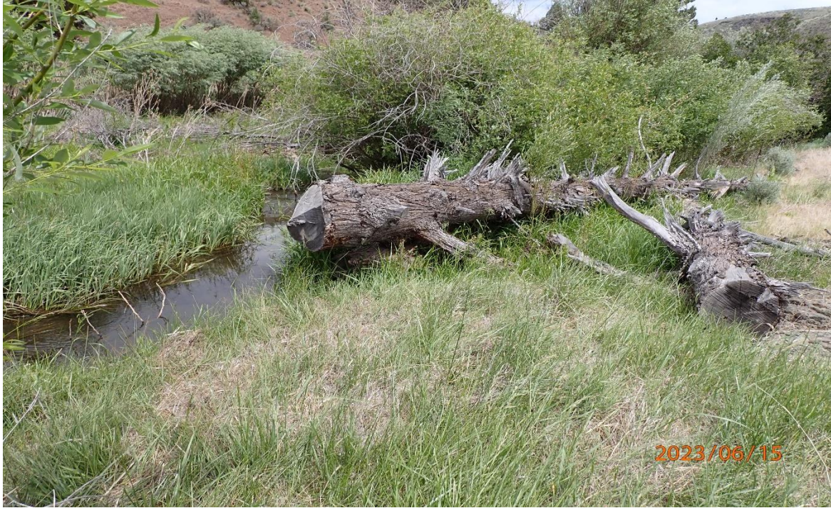
Above: Stream channel with large woody placement.
