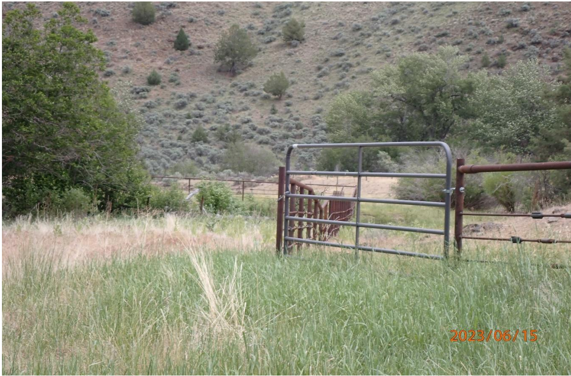
Below: HD riparian fencing installed, showing gate access.
