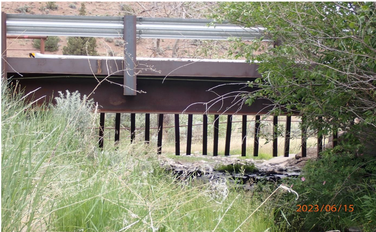
Below: Upstream, after bridge installation.
