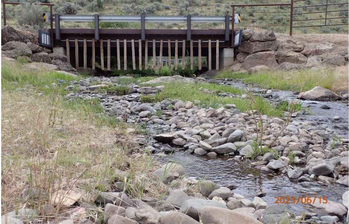
Above: After instream grade control riffles were installed.
