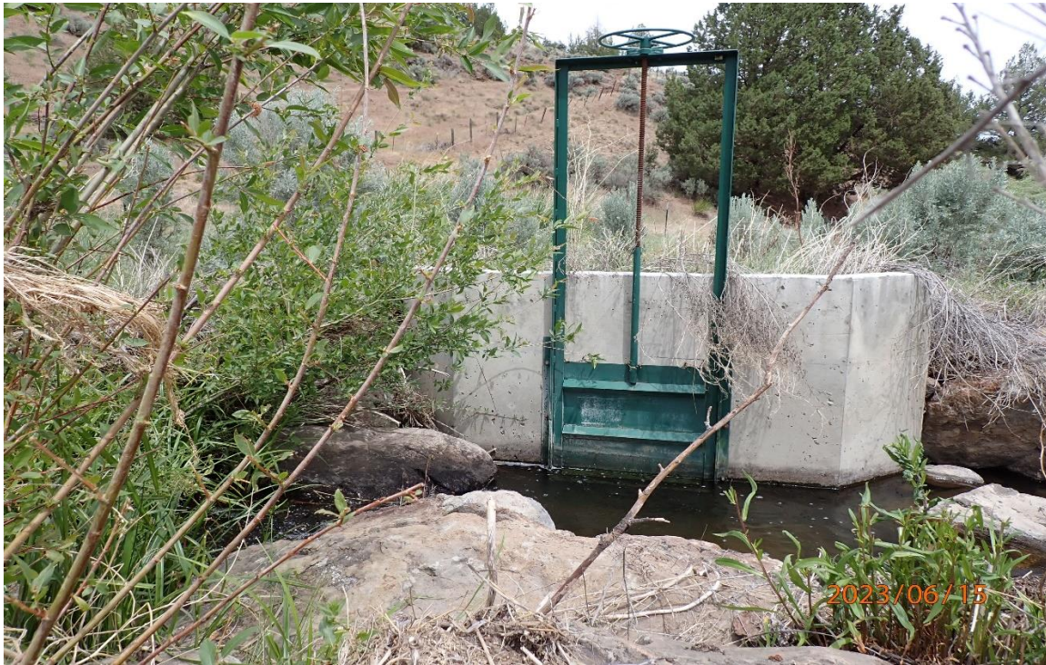
Above: New diversion structure.
