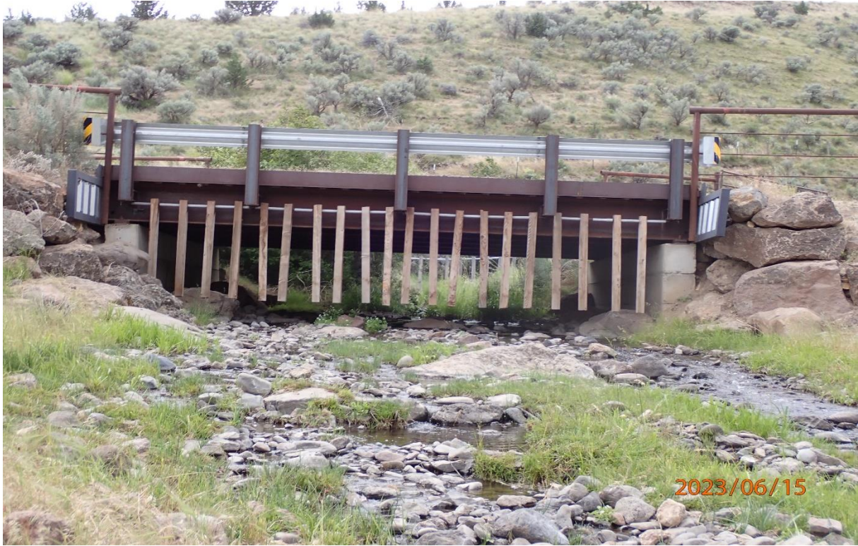
Above: Downstream, after bridge installation.
