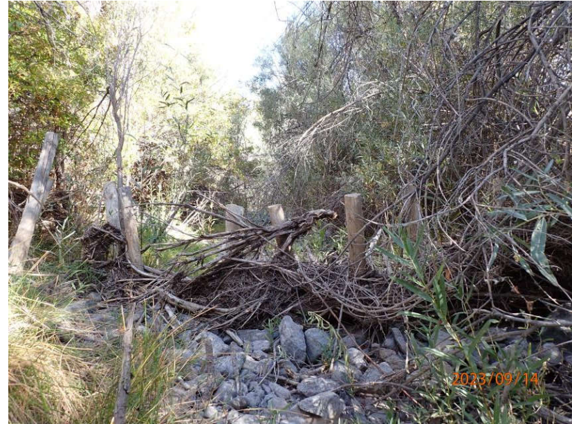
Rancher #1 (2023) BDA structure still established and capturing debris and sediment when surface water is present.
