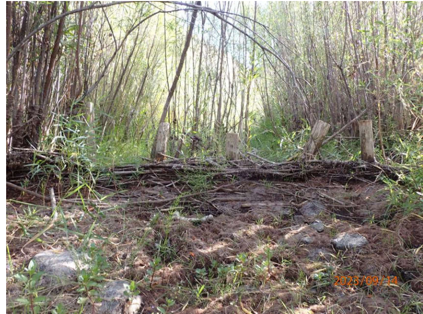
Beaver #4 (2023) BDA structure still established, capturing debris and sediment.
