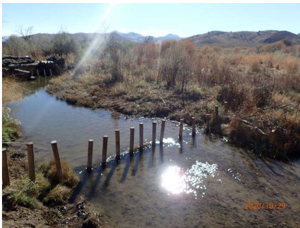
Above: Photo Point #24- View of BDA structures and large woody debris in the background.
