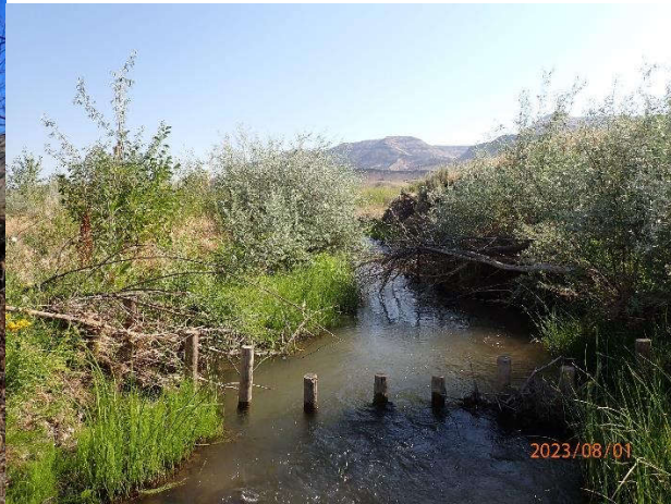
After: BDA structures with floodplain connectivity.
