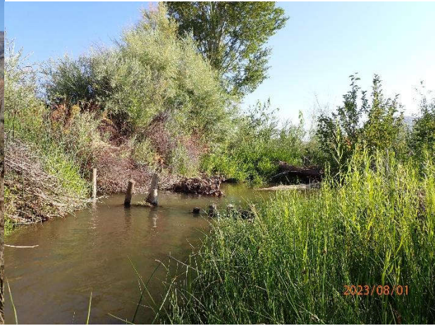
After: BDA structure silted in and large woody debris shifted with high flow, but still creating scour pool.
