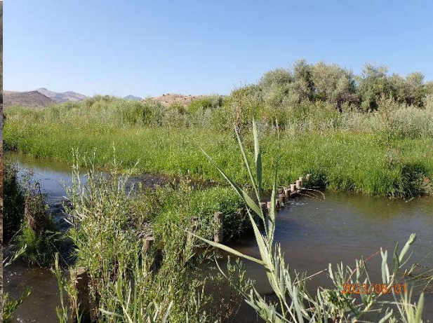
After: BDA still present and capturing debris.
