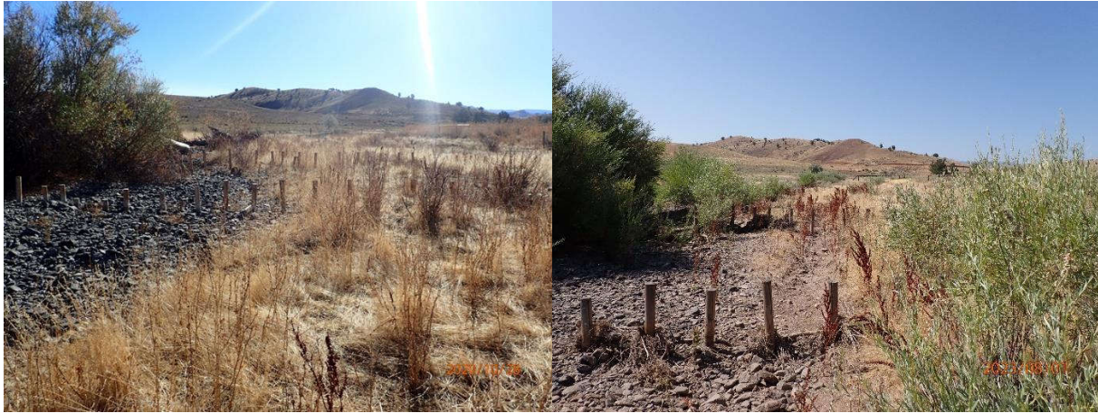
Above: Photo Point #5- Overview of BDA structures in Bear Creek.
