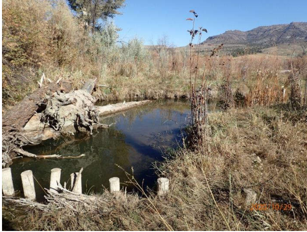
Above: Photo Point #37- Close up of BDA structure and large woody debris creating scour pool.
