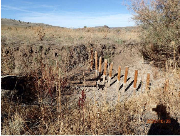
Above: Photo Point #7- Overview of BDA structure and large woody debris.
