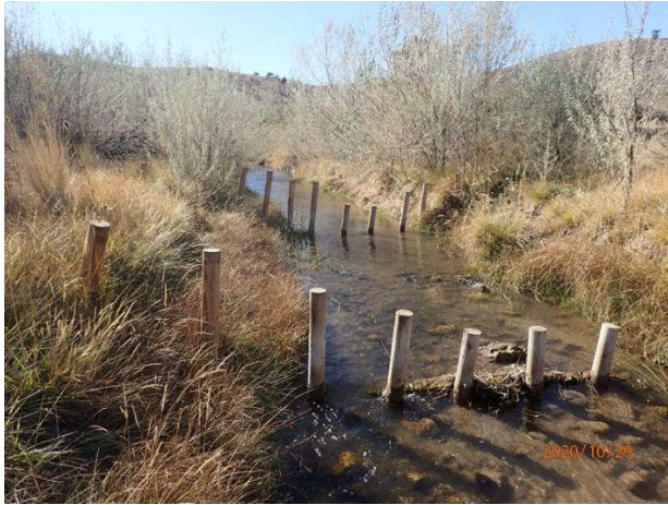
Above: Photo Point #33- Close up of BDA structures, riparian species, and vegetation.
