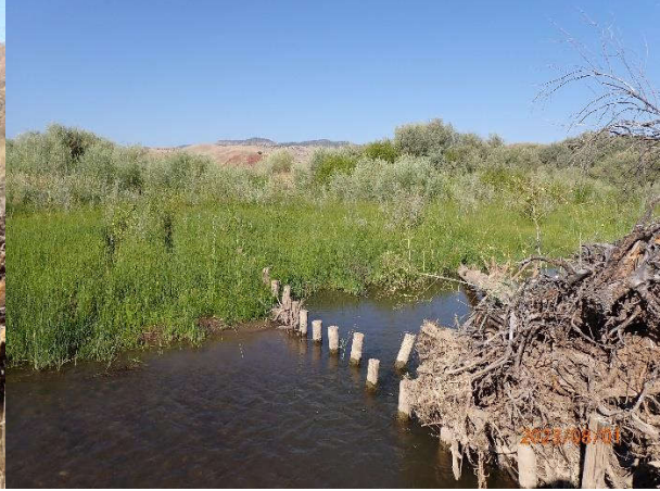
After: BDA structure still present in creek and floodplain.
