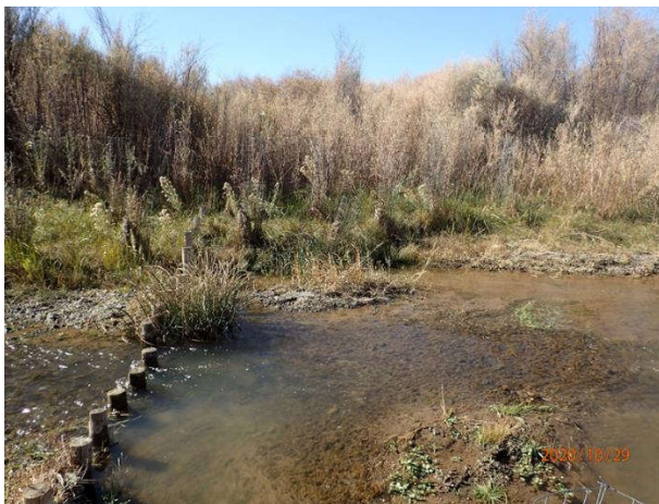
Above: Photo Point #28- Overview of BDA structure spreading water into the floodplain.
