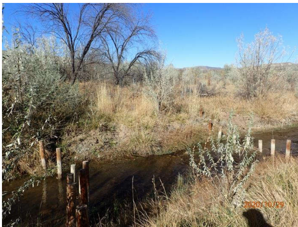
Above: Photo Point #30- Close up of BDA structures on Bridge Creek.
