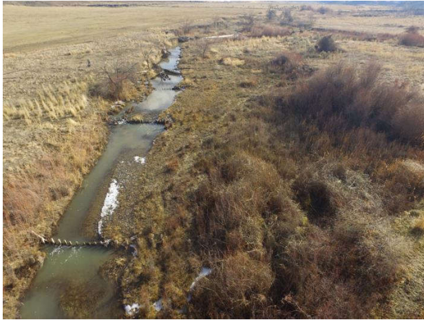
Above: Photo Point #42- Aerial image showing all project elements; BDA structures, repaired BDA structures, and LWD placement. Located near photo point 27.
