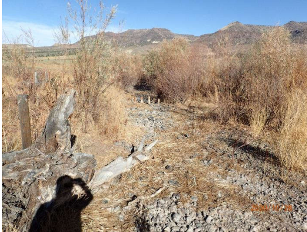
Above: Photo Point #13- Overview of BDA structure and large woody debris.
