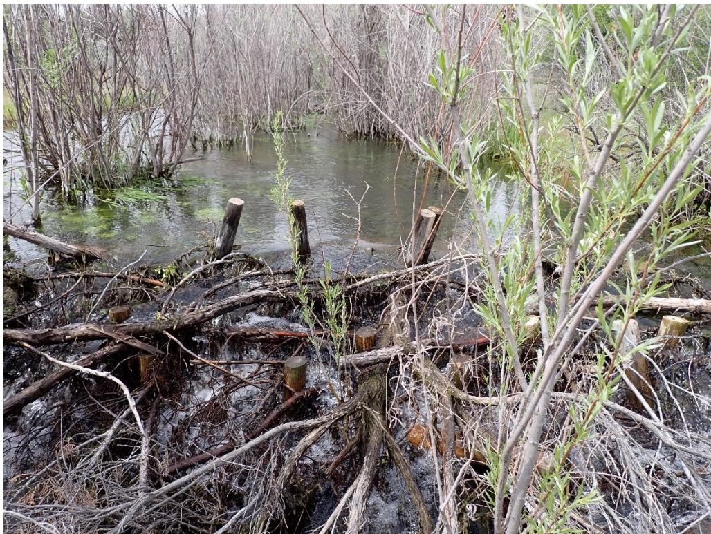
Below: BDA installed near the top of a riffle. Point #8
