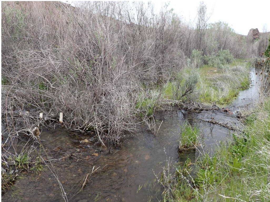
Below: View of structure #2 from different angle with engagement of side channel. Point #20
