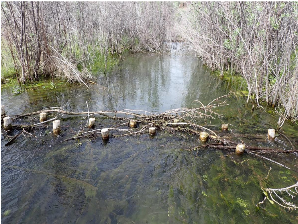
Below: BDA installed at the top of a lateral scour pool. Point #6
