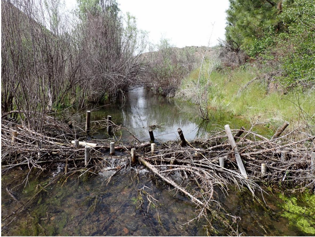
Above: BDA structure expanding stream bank and increasing pooling. Point #3
