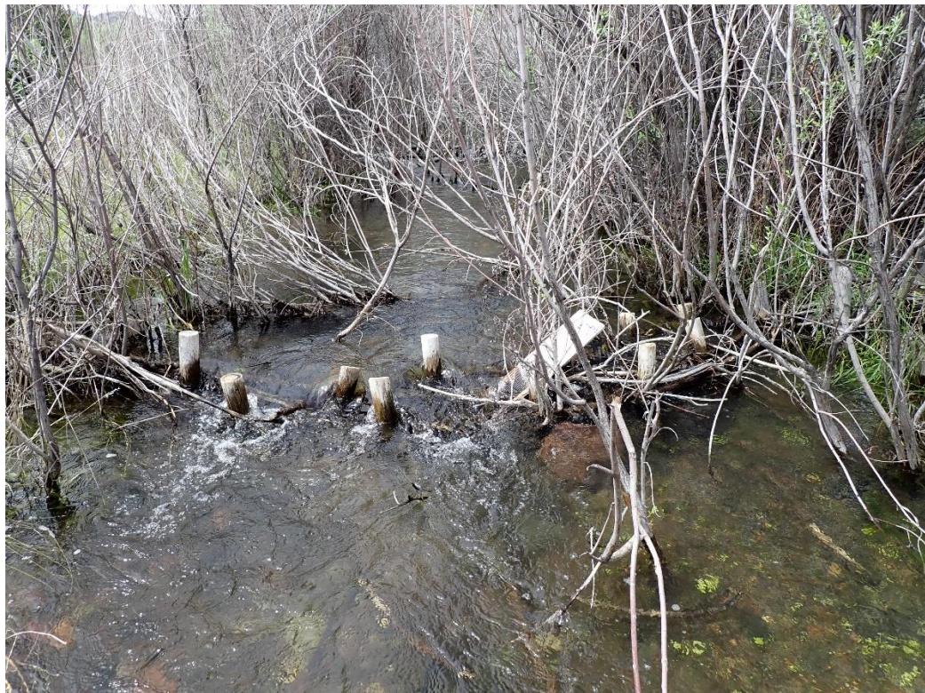
Below: View of another BDA structure at the bottom of a riffle. Point #18
