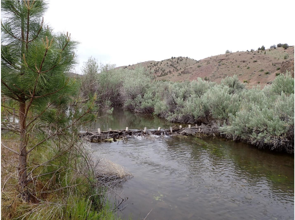
Above: Constructed BDA structure # 8 showing flood plain connection. Point #24
