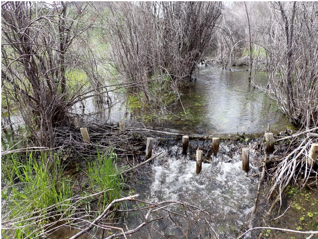
Below: BDA installed at bottom of glide. Point #16
