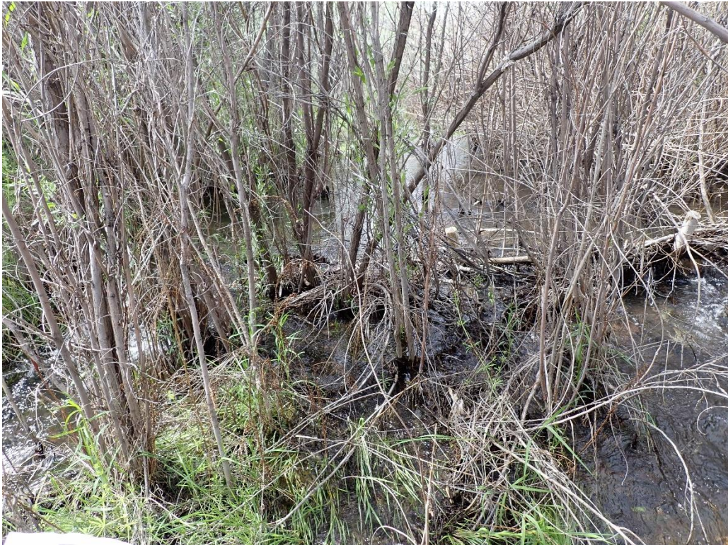
Below: Barely visible BDA installed at a glide. Point #10
