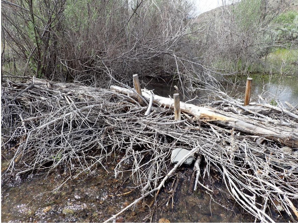
Above: A BDA installed at a glide. Point #11
