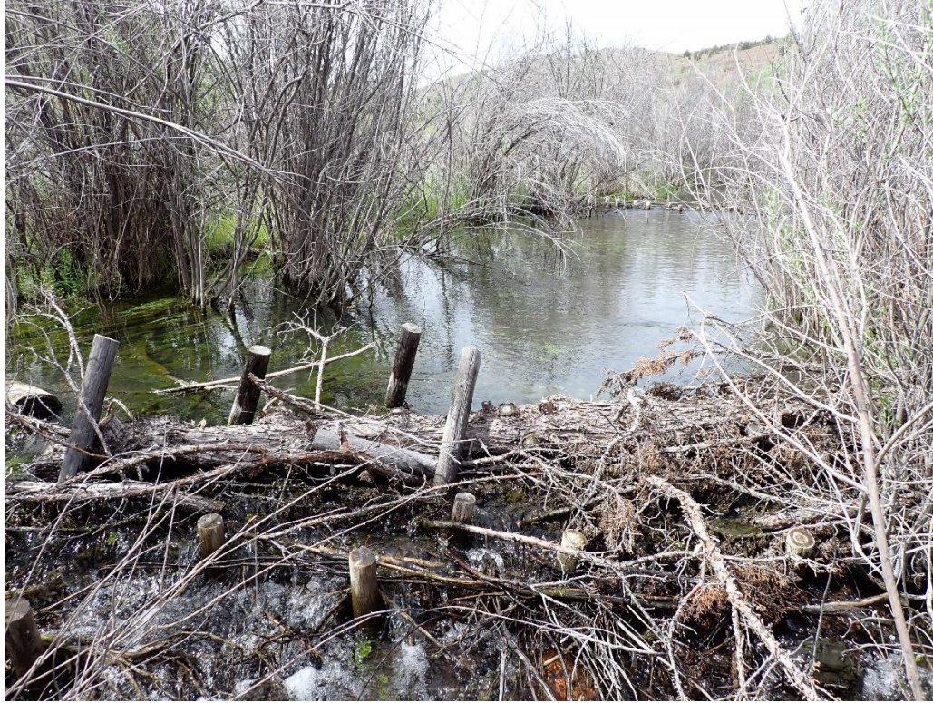
Above: BDA installed at the bottom of a lateral scour pool. Point #5
