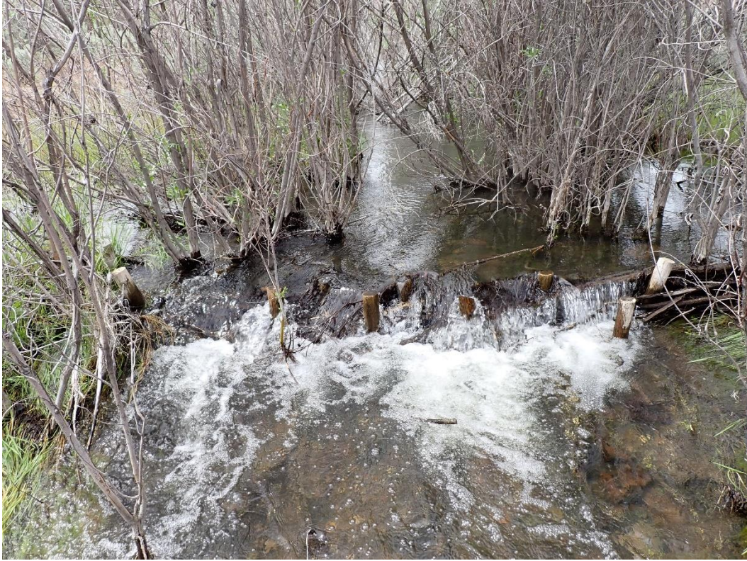
Above: View of BDA structure at bottom of a riffle. Point #21
