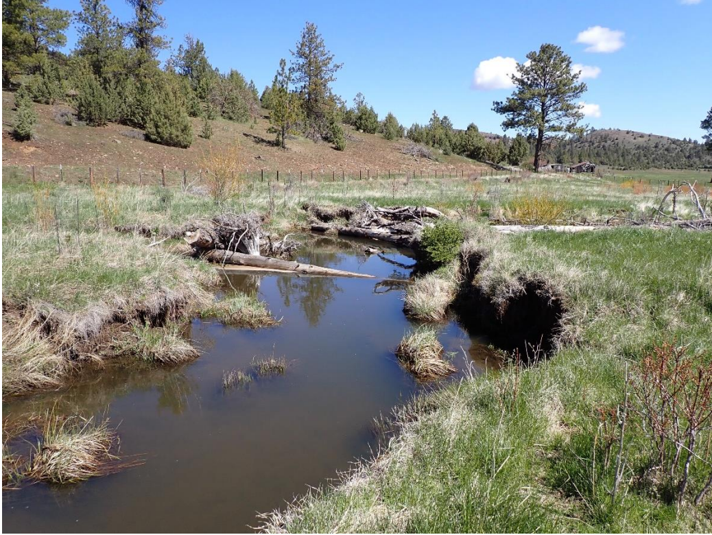
Above: Facing down-stream showing in-stream work with large wood material.
