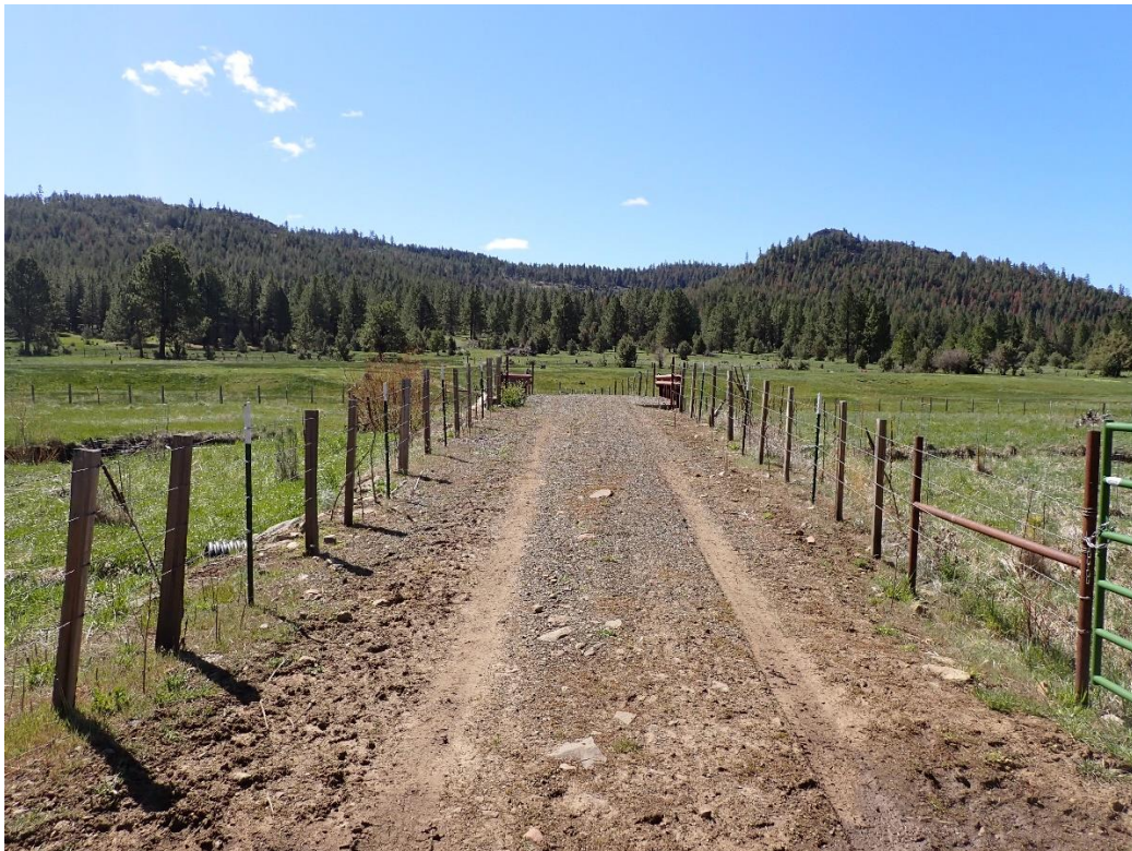
Below: North of bridge facing south showing CREP exclusion fence.
