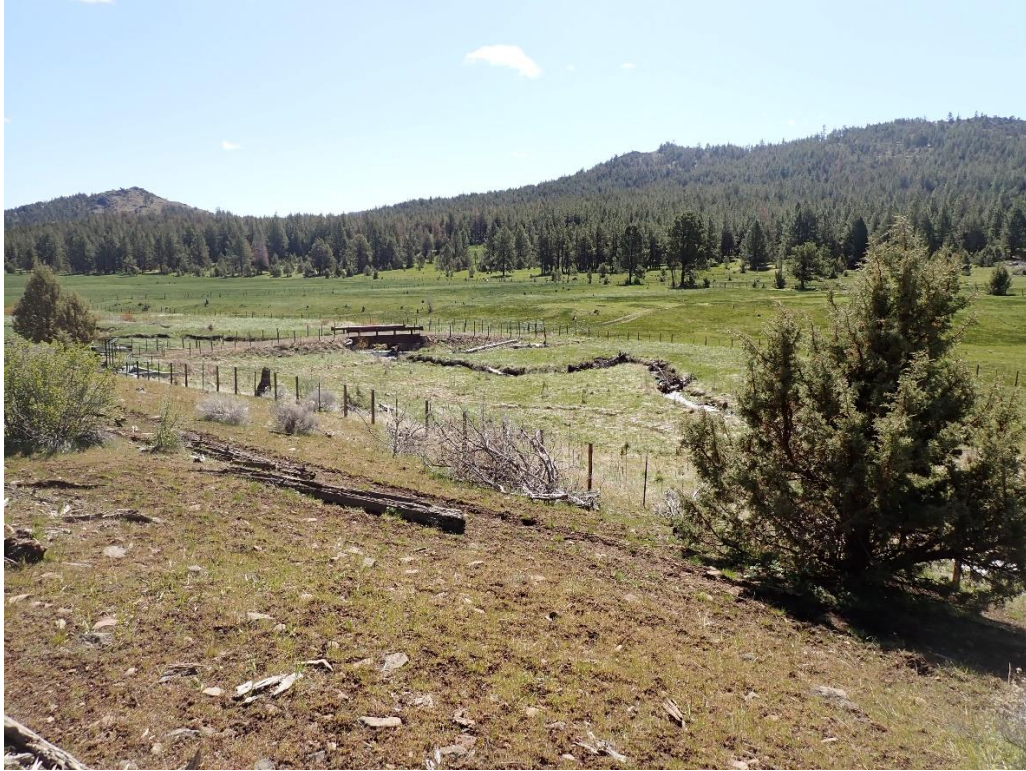
Above: Overview of Badger Creek diversion, bridge, and riparian restoration area.
