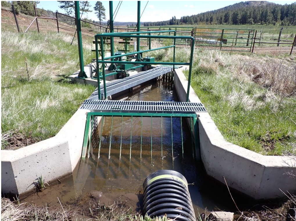
Below: View of completed fish screen not shown in final report.
