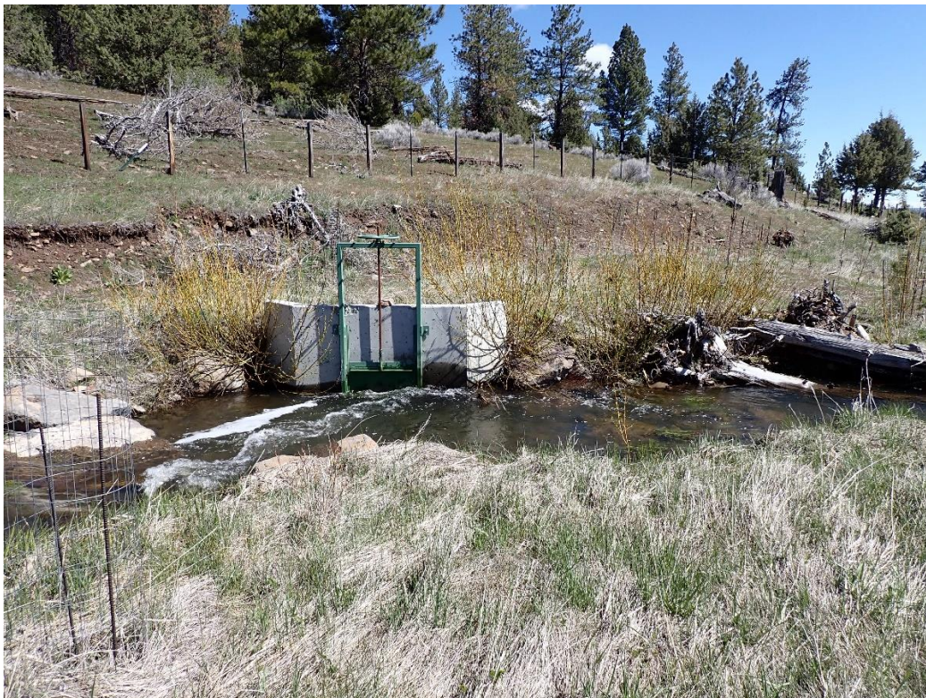
Below: Close up of new diversion and scour pool facing north.
