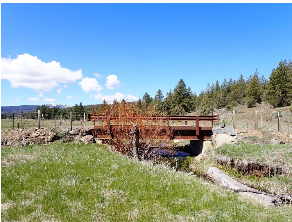
Below: Down-stream from bridge facing west showing completed project components.
