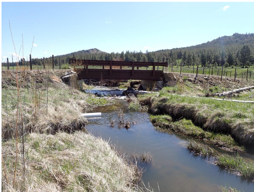
Above: Up-stream from bridge facing east. Showing fish return pipe.
